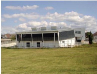
• Building a wholesale fish market in Poreč
