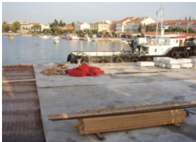
• Building a fishing pier in Umag
